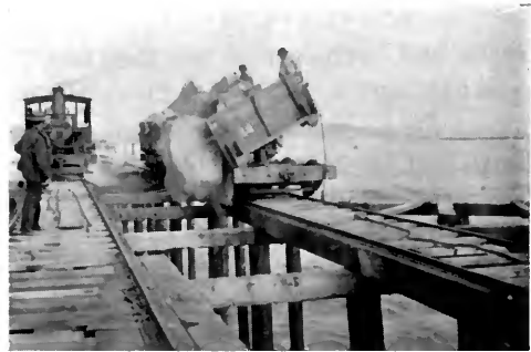
HYDRAULIC DUMPING CARS—NORTH JETTY.
